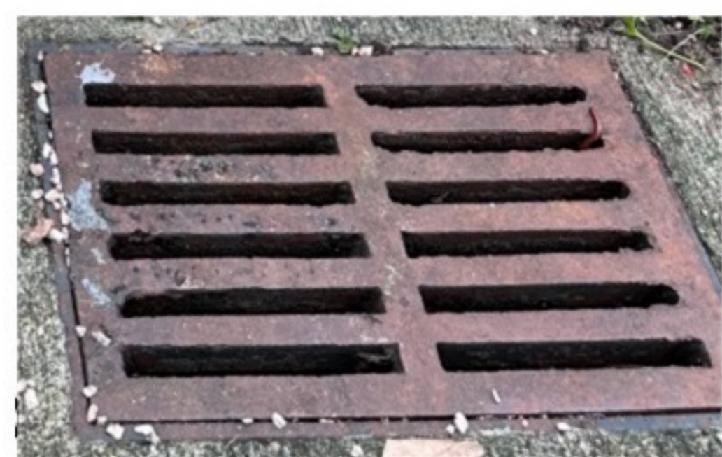
Drain outside farm on pavement
